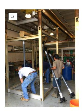
Train 2 – two cassettes and old membranes and hardware removed. Getting ready for rebuild
