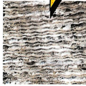
Old Refrigeration Coils
